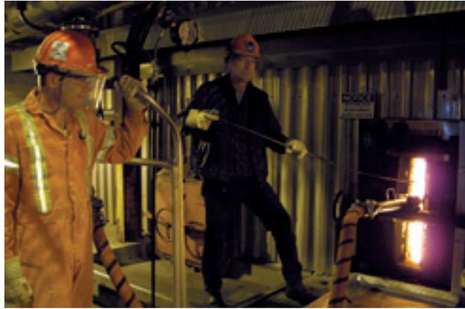
Dale Rietze and Victor Scott cleaning the black liquor nozzles in the recovery boiler. Black liquor is sprayed into the recovery boiler, atomizing it into small droplets that burn easily.
